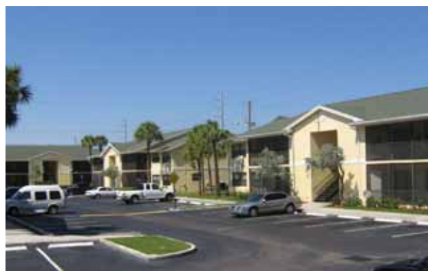
Caroma was chosen to conserve water at College Gardens Apartments.
